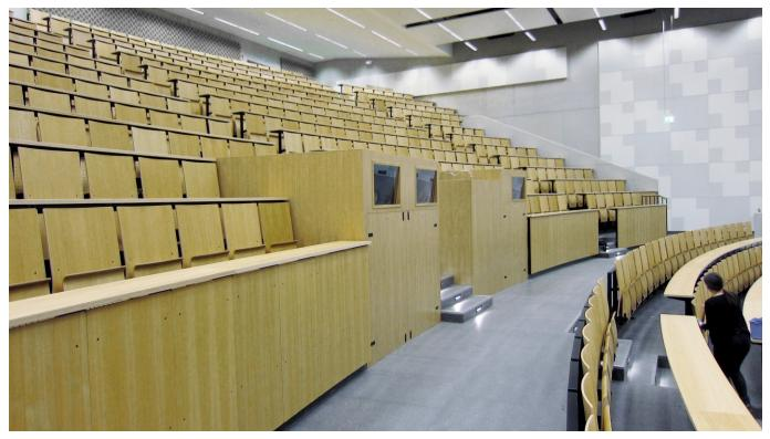
Here you see noise reduction cabins in a lecture room of a university. 3 independent projection systems (see the projection windows) were integrated in this environment. Projectors are build onto rail-systems to make lamp changes very fast. The carpenters work was very demanding, because of the curved shape of the seating.
