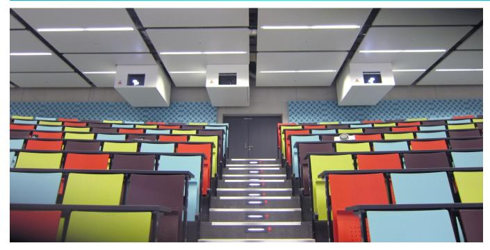
Three big xenon projectors have got perfectly designed soundproof housings. The heat outlet is integrated and interacts with the air condition. Each enclosure has an integrated lift. Servicing of the individual unit is no problem at all and can be done in table height.
